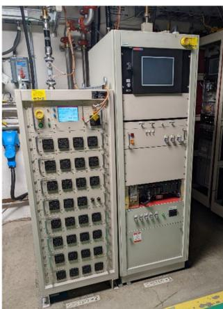
As installed for operations: new 10-kW SSA (left) and backup 3-kW tube amplifier (right)
