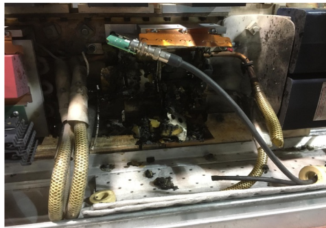
Transistor failure due to transformer saturation
