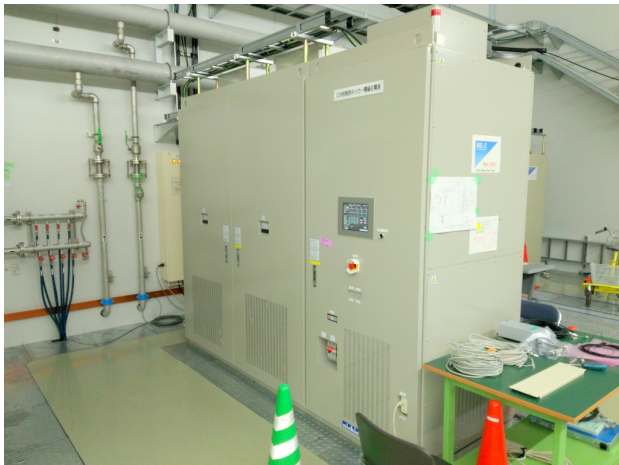
SiC power supply (60 Hz, 1 kV-299 A)
