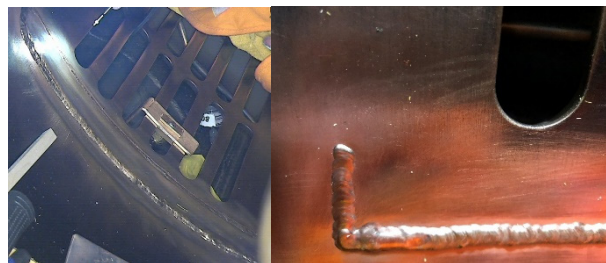
Figure 6: Welded patch (left) and heat induced crack (right).
