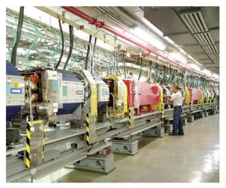
Figure 2: Photo of the APS storage ring within the accelerator enclosure [21]. Prominent in this image are the flexible tubing (aqua) serving individual accelerator components, connected to the water manifold at the ceiling. The fire sprinkler piping (painted red) is also visible along the ceiling. [Adapted under CC BY-NC-SA 2.0 license from Ref. [21].]
